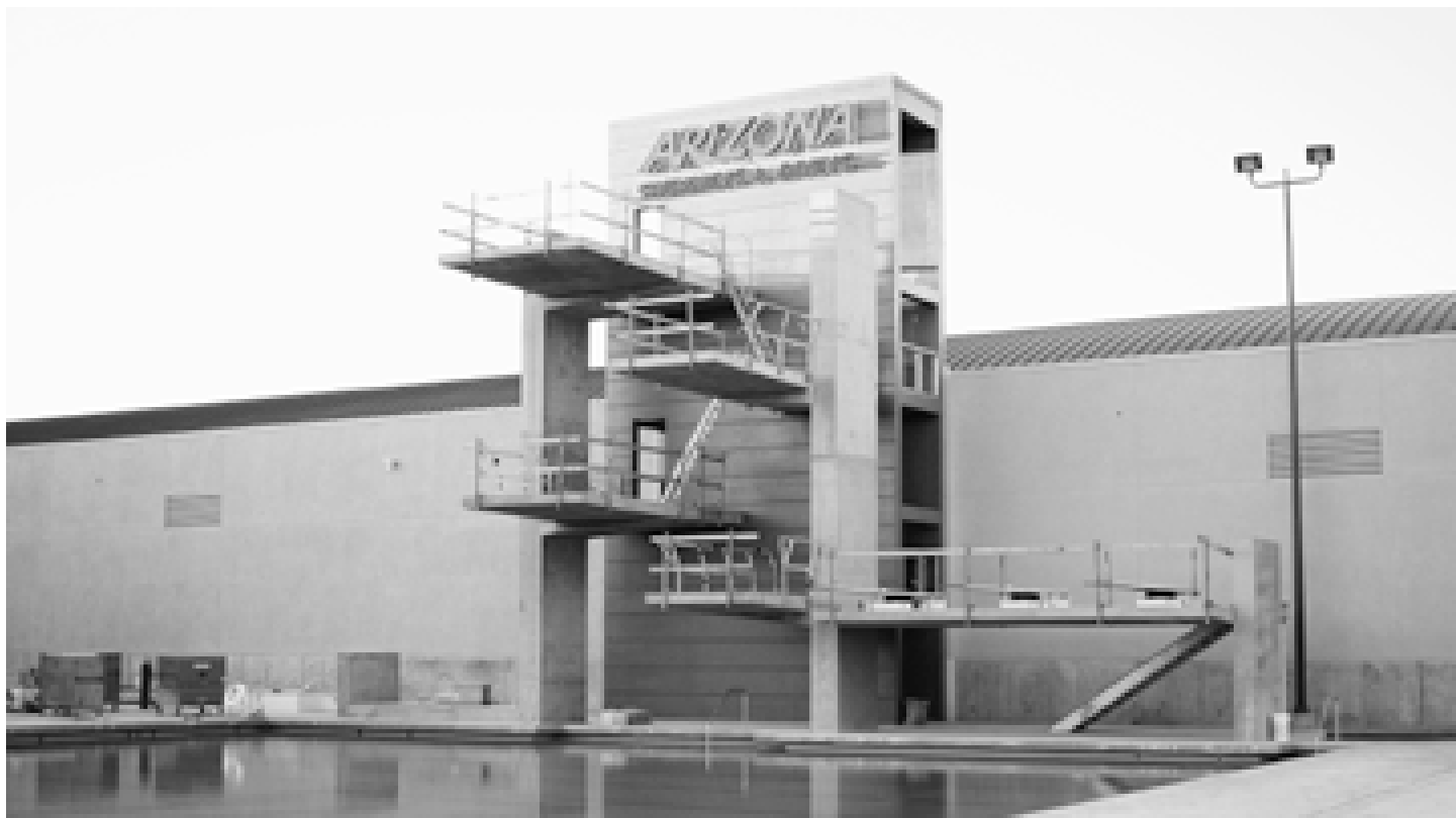
The new diving tower features two 1-meter and three 3-meter Maxiflex Model "B" springboards on concrete short stands as well as platform heights of 3, 5, 7.5, and 10 meters, each with Rough-Tex surfacing.
